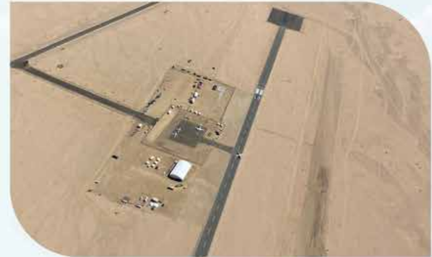
Saudi Aviation Club Airport in Al Madinah (Al Mindassah) 43 KM North of Al-Madinah
