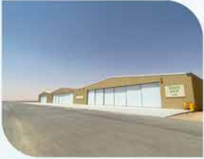
1800sqm SAC Parking Hangar
